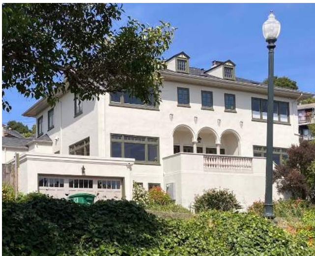
Renaissance Revival, Arlington Ave., 1919, James W. Plachek
