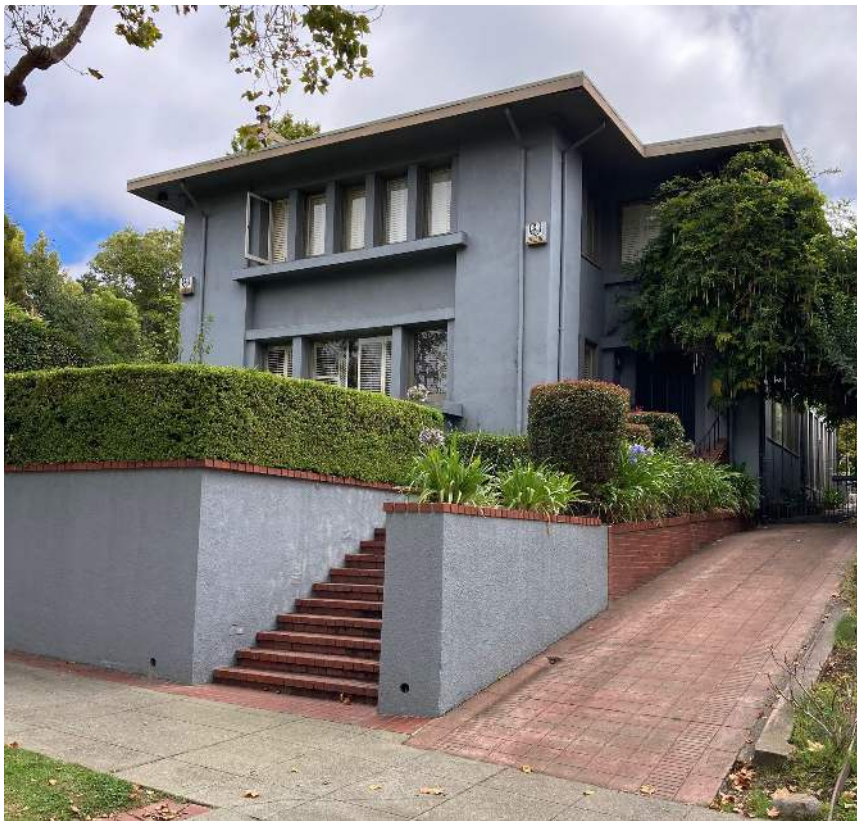
Prairie Style, Mariposa Ave., Olin S. Grove, architect, 1911
